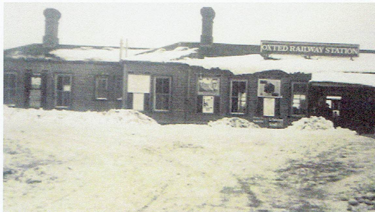
Oxted Railway Station, c.1910
